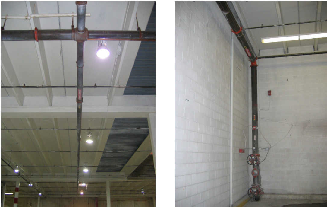
Figure 1. Typical Sections of Fire Sprinkler System
